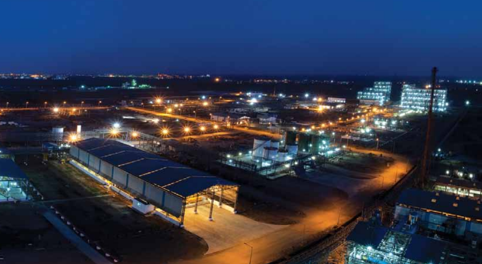
Chemical Complex, Dahej, Gujarat
