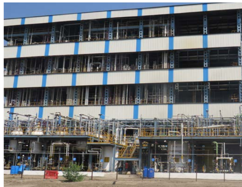
Agrochemical AI manufacturing plant
